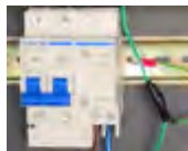
N1042826 Current Protection Switch
